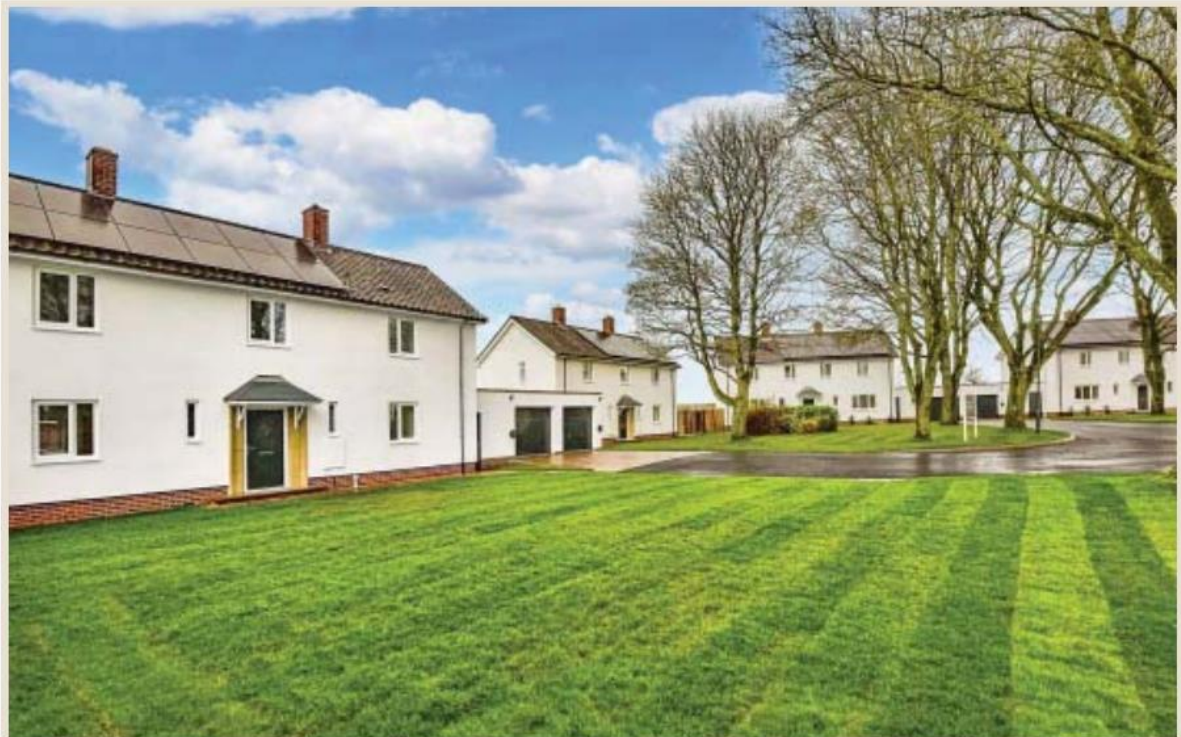
The newly renovated former MoD homes in Devizes
